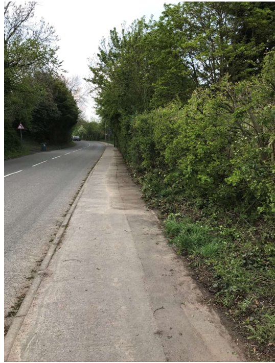
Melton Road - After
