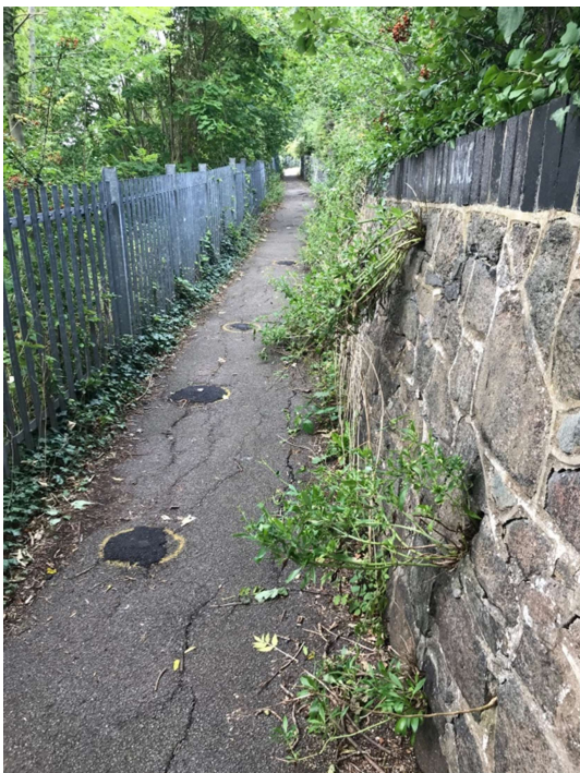
Before – lots of low laying growth along the path
